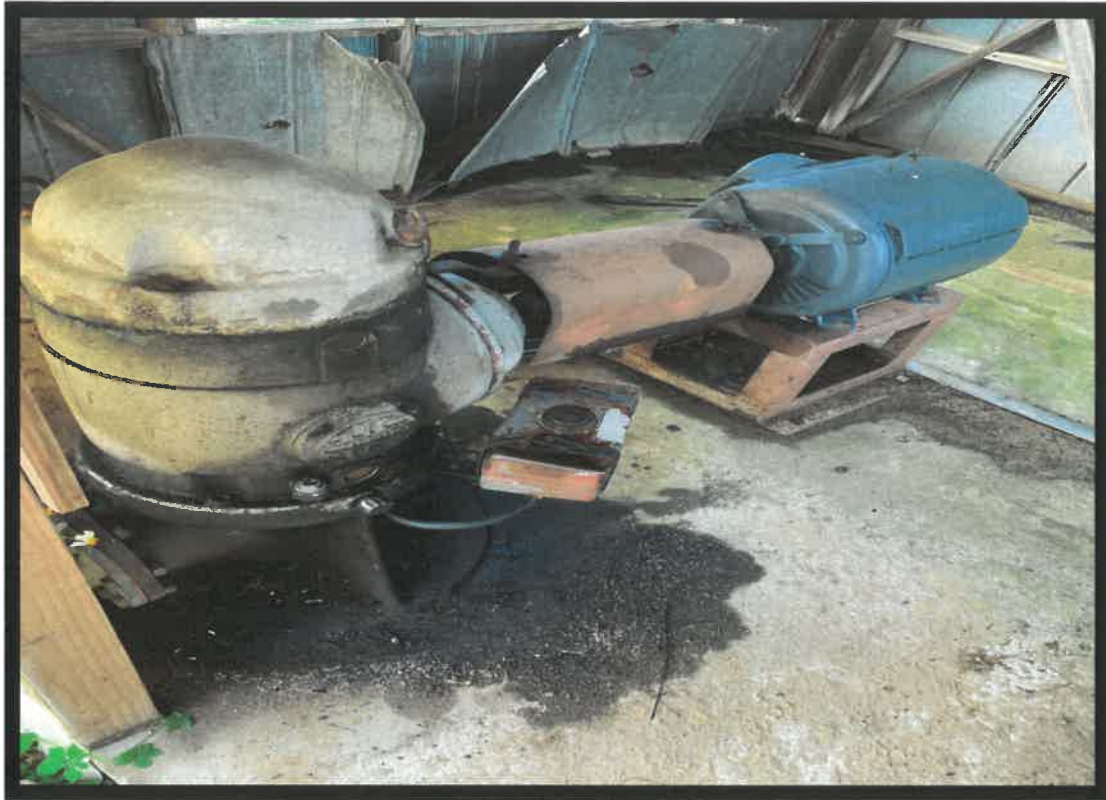
Photo 7 – Irrigation Pump inside Pump House.
